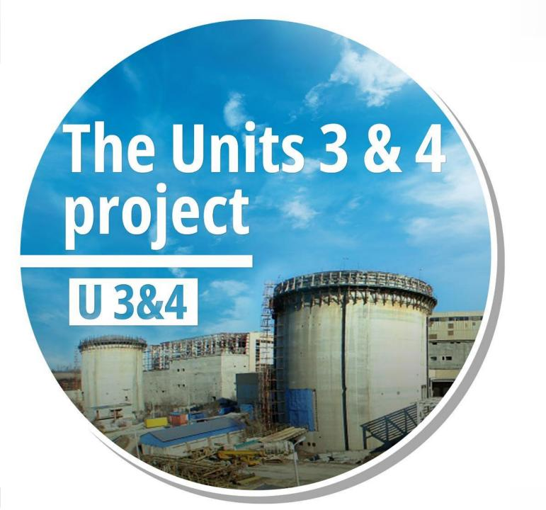
CANDU UNITS 3 & 4 PROJECT AT CNE CERNAVODA - consists in the completion of the construction and commissioning of 2 units of at least 724 MWe installed each, with annual electric energy output of more than 10.5 TWh, each.
