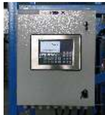
Design, fulfilment, delivery, mounting, calibration - Large bags weighing and bagging system. Capacity from 500 up to 1500kg, accuracy 0,1%. ALUM Tulcea; BCG Ploiești; Fertil Plant Constanța - Romania
